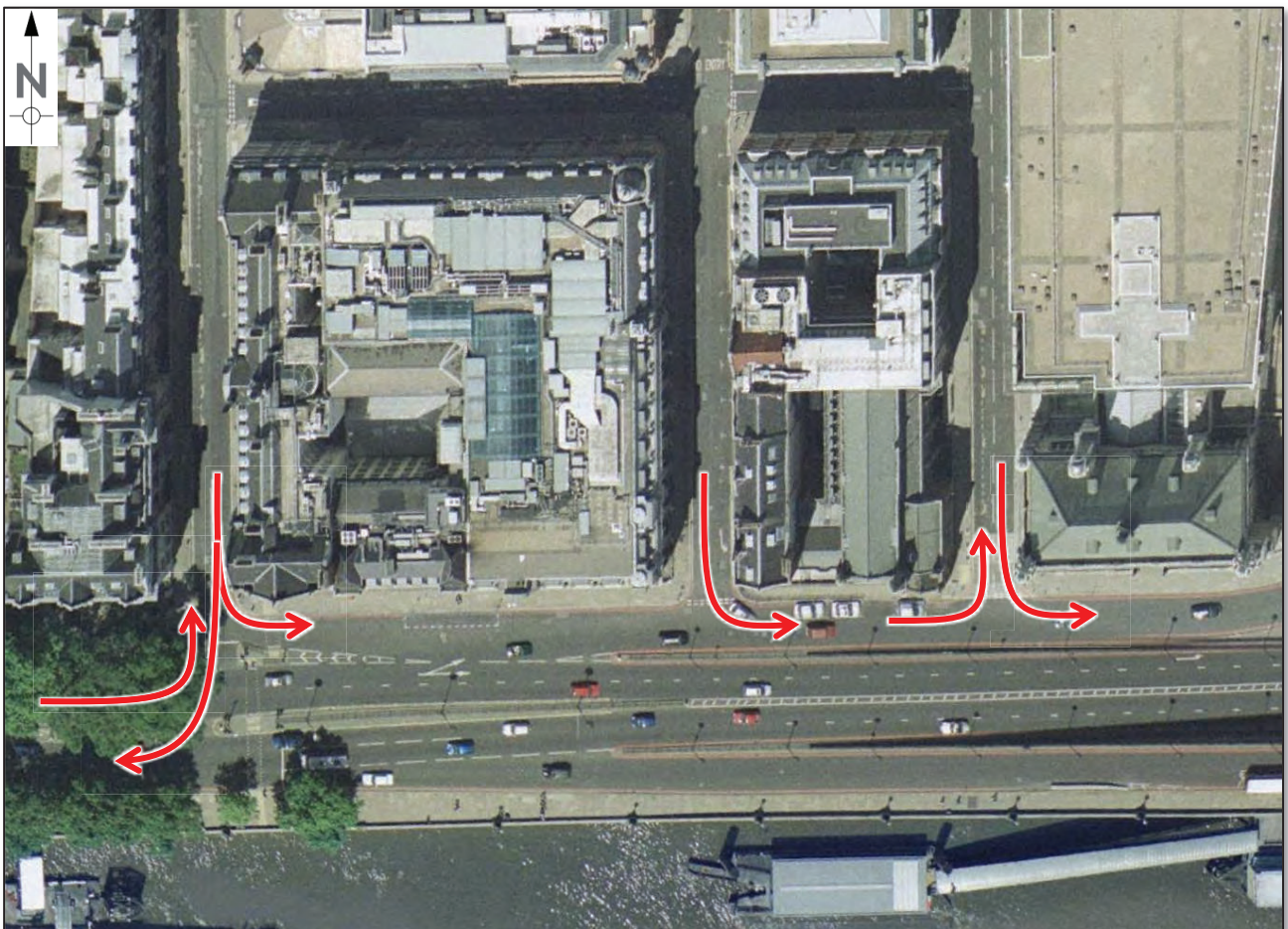
Figure 5-1: Access between Whitefriars area and Victoria Embankment (pre-2005)
